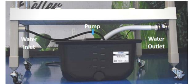
5.1 Place the reservoir under the Bottom Layer in between the bottom legs. Place the lid with the opening towards the front. Connect the drain hose to the water outlet then tighten the clamps. Do NOT over tighten. Place the loose end of drain hose inside the reservoir through the lid opening.
